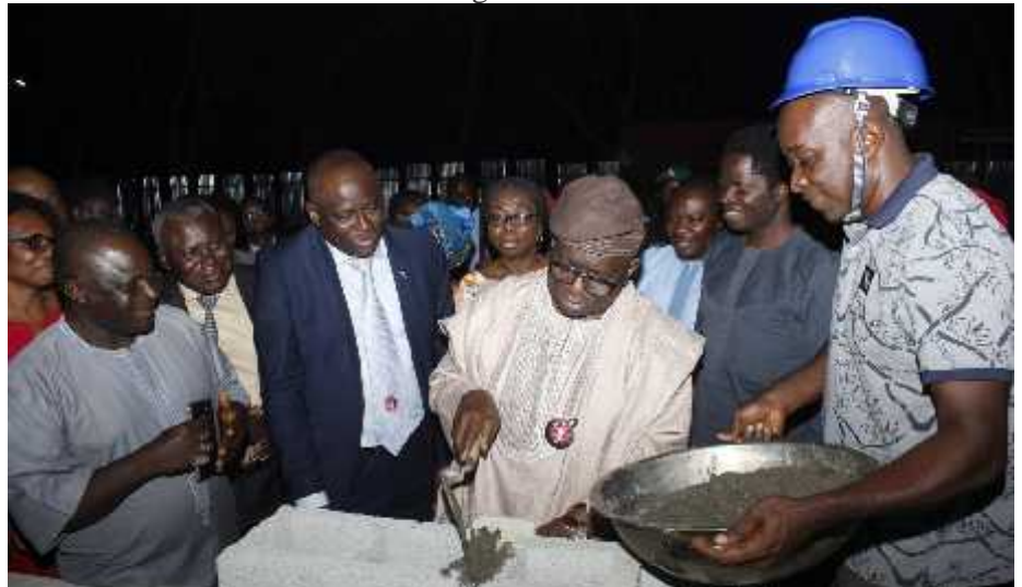
Minister of Health, Prof. Isaac Adewole laying the foundation for the UATH Accident & Emergency Extension.
